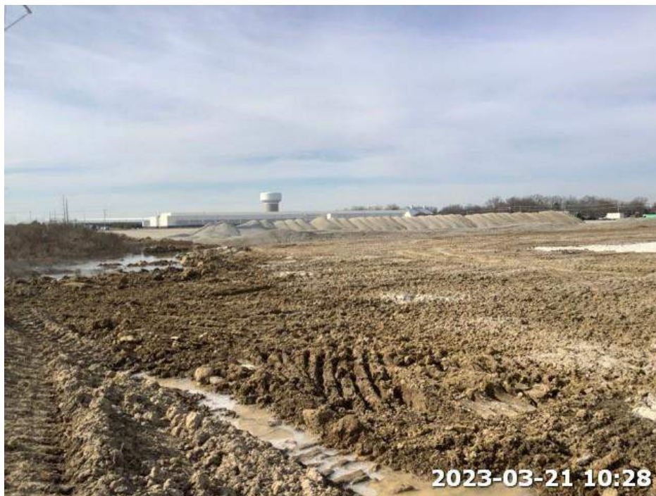
Photo 2. View of previously delineated Wetland 1 area. Photograph taken facing southwest.
