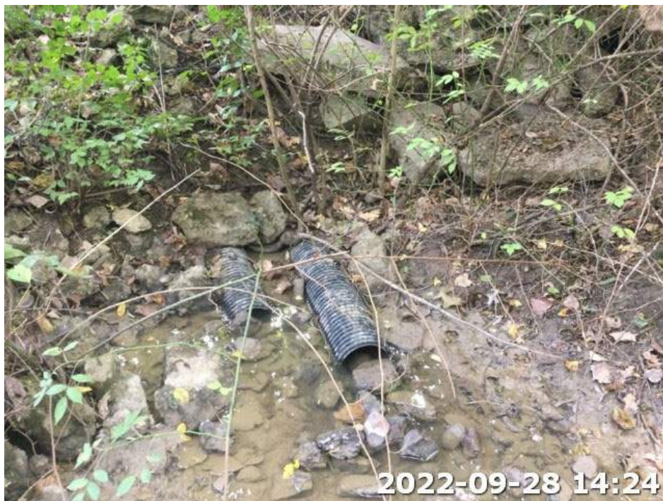
Photo Location 7. View of typical culvert. Photograph taken facing east.
