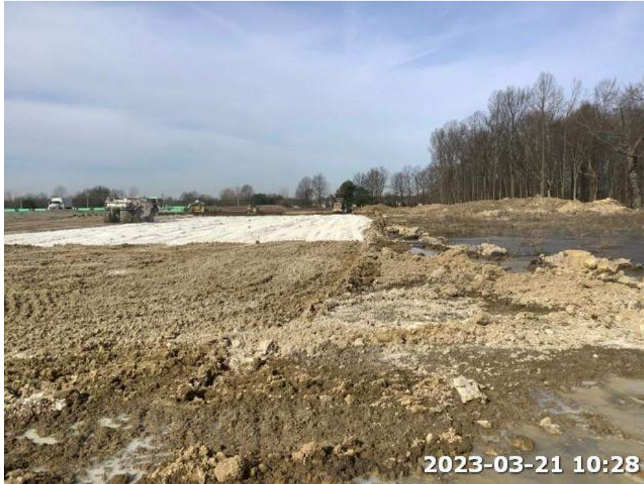
Photo 3. View of grading activities in northeast corner of the Project area. Photograph taken facing west.
