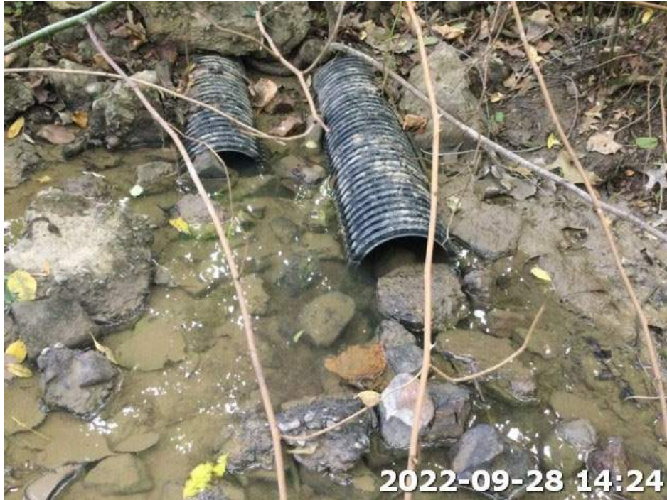
Photo Location 7. View of typical culvert. Photograph taken facing ground.
